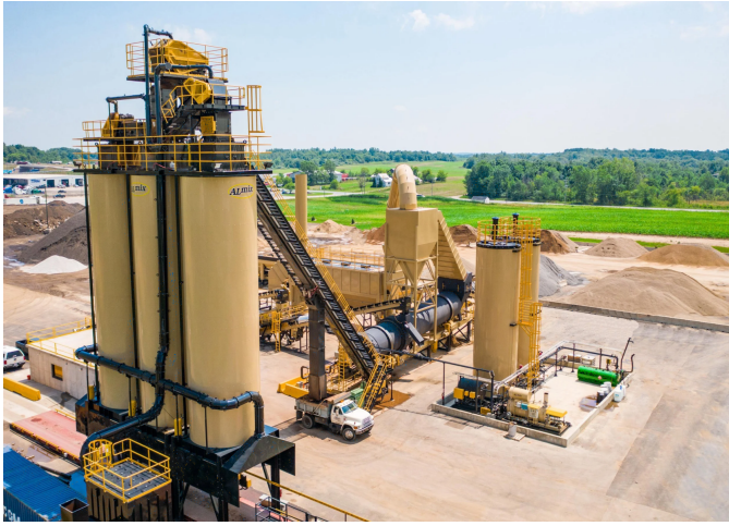
□ Asphalt Plant Demo Report
