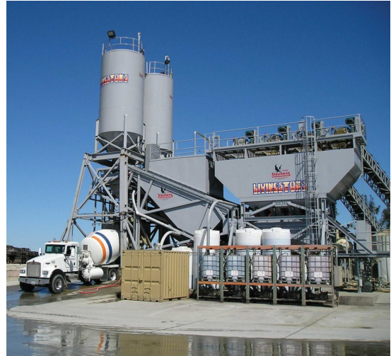
□ Ready-Mix Plant Demo Report
